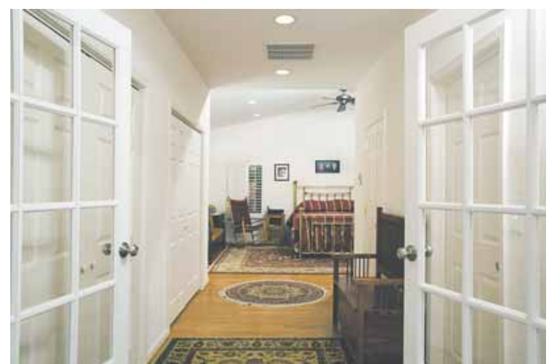
The louvered door on the right is for the family's Irish setter, who exercises in the side yard. All doors are at least 32 inches wide and have a 90 degree clearing width.
