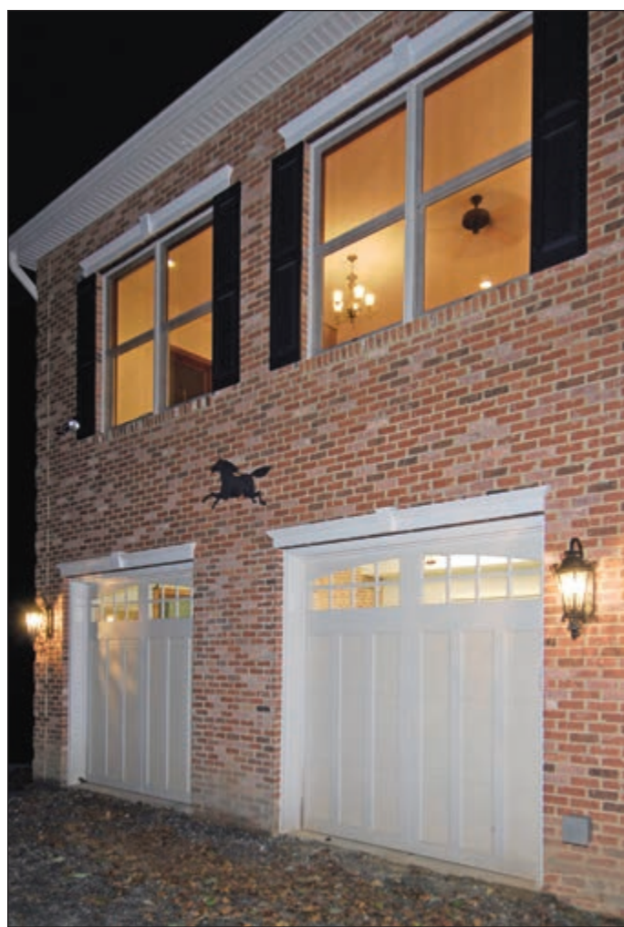
The now west-facing two-car garage is accessible through an interior door that parallels the archway. The addition's second floor accommodates a guest suite, the laundry and a substantially enlarged master bathroom suite.
