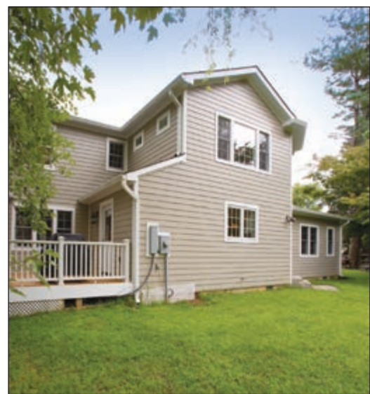
After opening up the existing home's rear elevation, Michael Nash added a 12-by-24 two-level addenda in the middle of the rear elevation and one level hyphen linking it to the rear of the garage. Decking and a screen porch complete modification. The entire exterior has been re-sided in Hardiplank.
