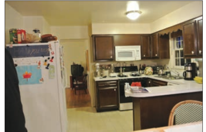
BEFORE: The footprint of the home's original galley kitchen was incorporated into a substantially enlarged "open" plan. To connect the new addition to the existing house, remodeler Michael Nash removed 22 feet of the rear elevation, supporting the second floor with a steel beam mounted on vertical supports.
