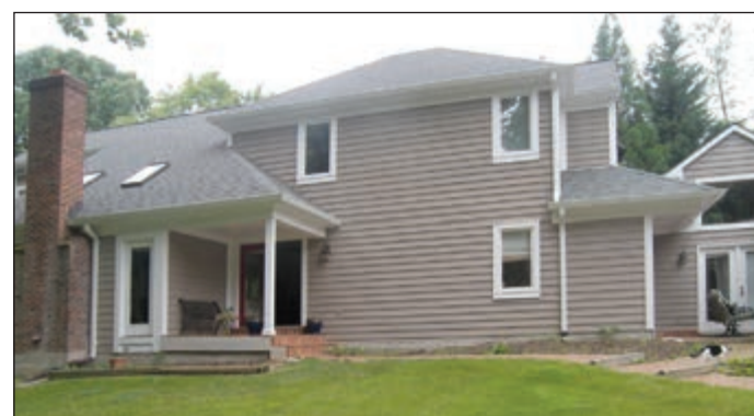
Before Exterior Front elevation
