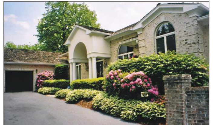
BEFORE: Assuring that the structural supports of a 15-year-old three-car garage could support the weight of a 1,110-square-foot "pop up" was a primary engineering consideration.
